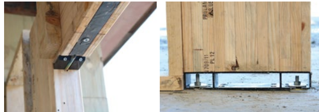
Knee Joint showing threaded rod Base plate attached to concrete
